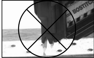
INCORRECT Placement of nail
